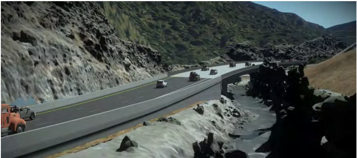
C-3: EB wall that you need for grade difference to get to Bridge N (visible wall seen from creek, Greenway, and US 6th)
