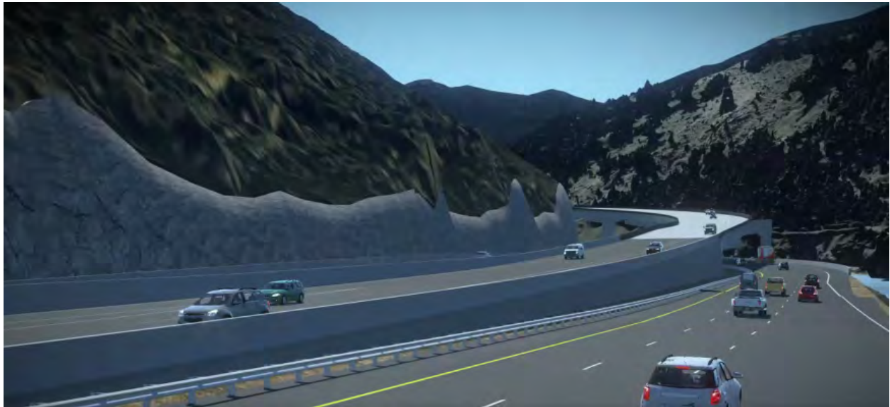
C-1: wraparound wall for where Bridge M (seen on right) lands (west abutment); very visible
