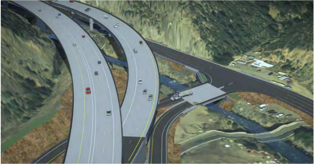
C-11 (north side) & C-12 : Abutment walls near bridge P & G (interchange at US 6); similar to bridge 241; C:12 wall along greenway trail that covers the grade difference for trail to get under Bridges P & G- likely to change to a grading solution versus a wall, more to come
