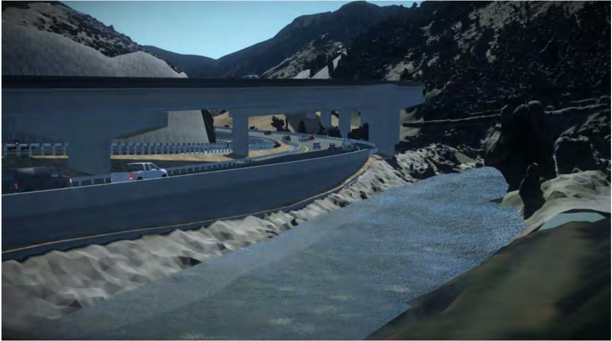
C-2: EB underneath bridge M, adjacent to the creek
